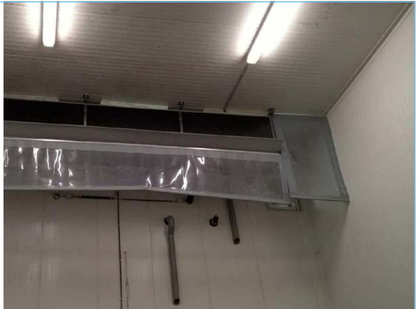
Flaps to improve ventilation in cooling
